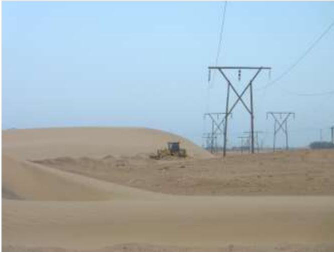
Figure 11. Mechanical excavation of sand dunes along the C14 road. Photo by Mattias Bovin (2010)
