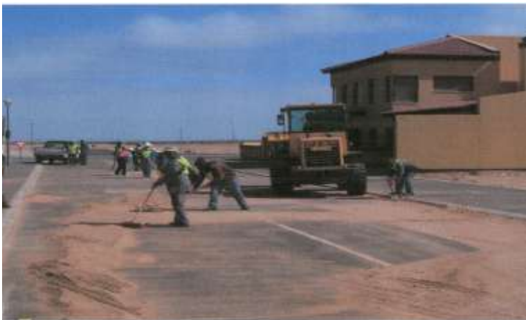
Figure 6. Sand removal after a sand storm (Louw, 2010)
